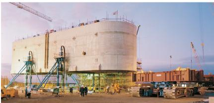
Split-Flow® pumps used for heavy lifting with strand jacks eliminate the need for cranes. In this application, PF3000 Series pumps with eight outlet ports replace flow dividers, providing increased output flow accuracy and consistent synchronized movement.
